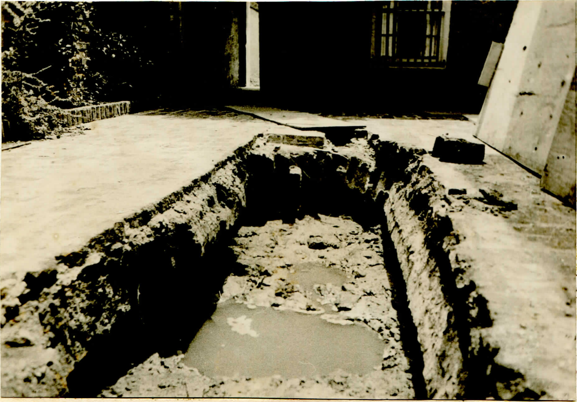
Figure 9. The cistern in back of the main building at 33 Broad Street.
